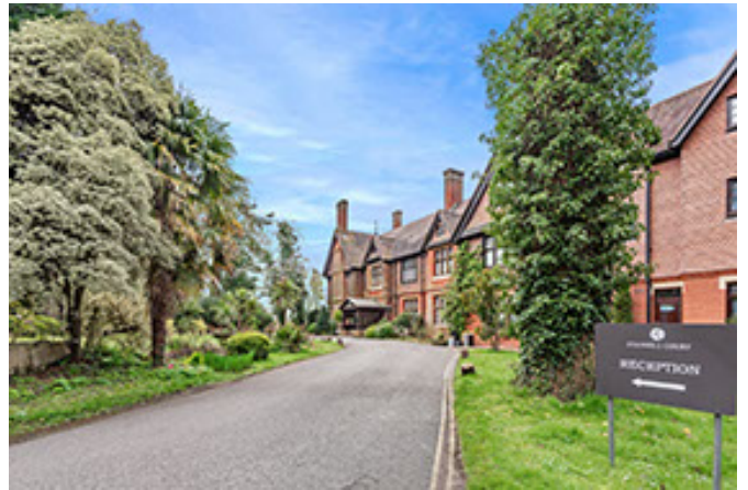
IMP Ref 3 Charlwood, Stanhill Court Hotel, Stan ...
