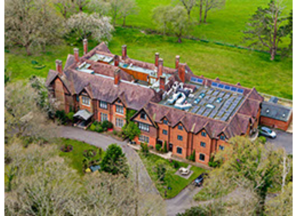
IMP Ref 3 Charlwood, Stanhill Court Hotel, Stan ...
