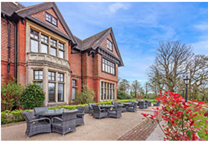
IMP Ref 3 Charlwood, Stanhill Court Hotel, Stan ...
